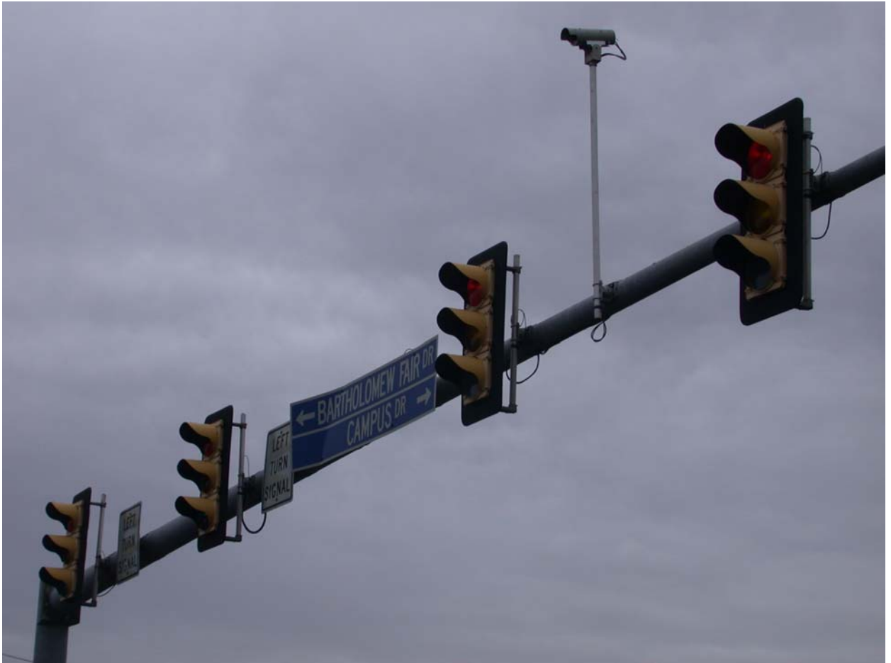
Figure 2: TYPICAL VIDS CAMERA INSTALLATION
