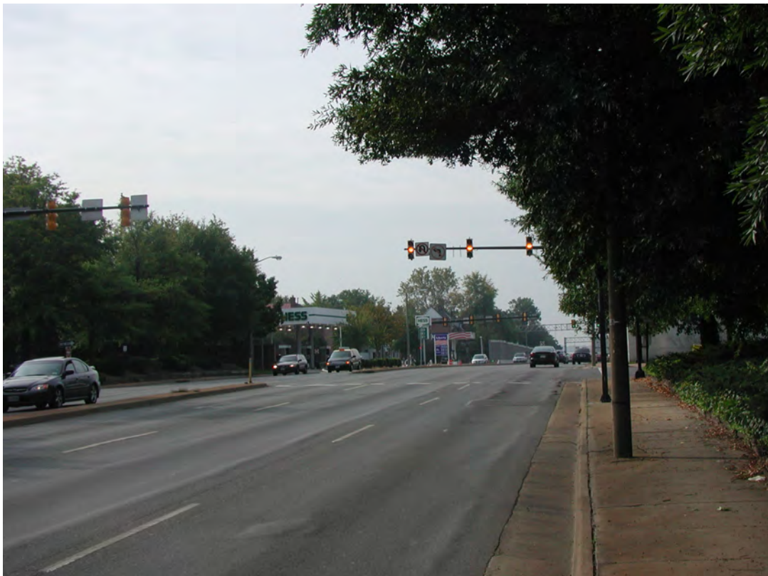
Looking south on Route 1 at Gibbon Street
